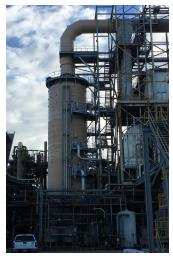
The lower section of the column treats quenched flue gas from an existing quencher and extracts heat into circulating cooling water so that the heat picked up is delivered via heat exchange to a number of locations that would require external heating otherwise. The entering wet gas is cooled and water condenses from it. The lower section also captures solid ash material coming from the boiler and removes it with the condensate created so solids level do not overload.
